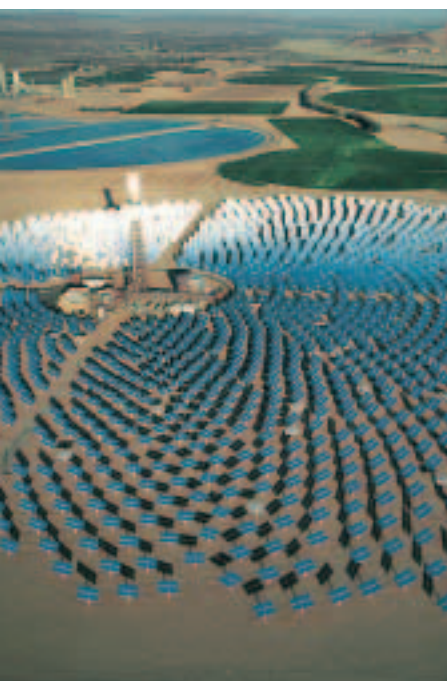
Figure 26-11 A power tower is surrounded by banks of solar panels that reflect and concentrate sunlight onto the tower, where the sunlight is collected and stored in batteries.
