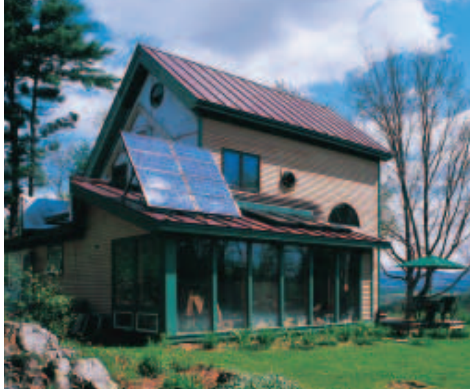
Figure 26-9 This house incorporates both passive and active solar heating in its design. Deciduous trees help block the Sun in the summer to keep the house cool. In the winter trees lose their leaves, allowing the Sun to warm the house directly.
