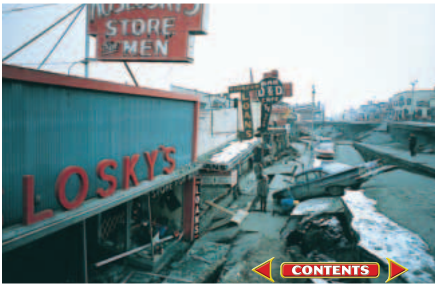
Figure 19-12 The damage shown here was caused by an 8.6-magnitude earthquake that struck Anchorage, Alaska in 1964.
