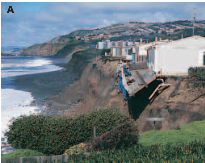
Figure 16-8 Shore erosion during a storm undermined the cliffs on which these houses were built, along the coast of Pacifica, California ( A ). The ocean has eroded the beach near Galveston, Texas, to the extent that the bases of telephone poles along a beach road now are under water ( B ).
