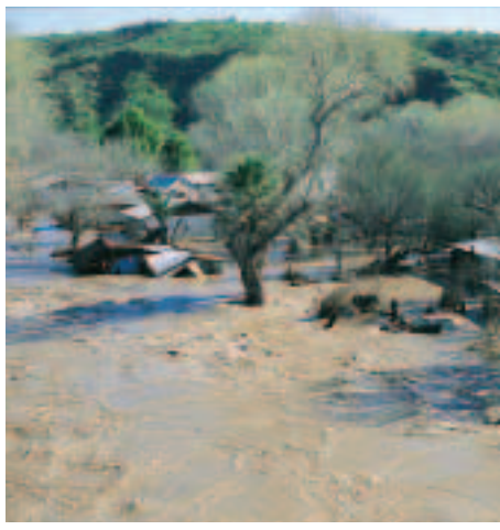
Figure 13-7 This rural community was devastated by a flood in Arizona.
